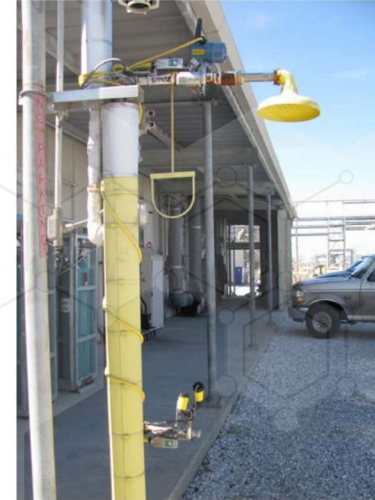
Figure 10: Adding a Rosemount 702 Wireless Discrete Transmitter can tell the control room which safety shower or eyewash station has been activated.
